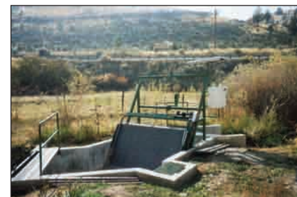
Hydrolox engineered polymer screens are lightweight enabling the solar power operation. The Hydrolox traveling screen pictured here is located in a remote location and is rotated using solar power.
