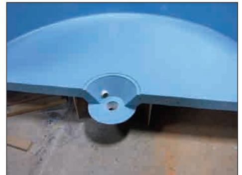
Tank Drain Cross Section
