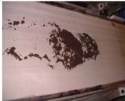
Add some flocculated sludge on the belt.
