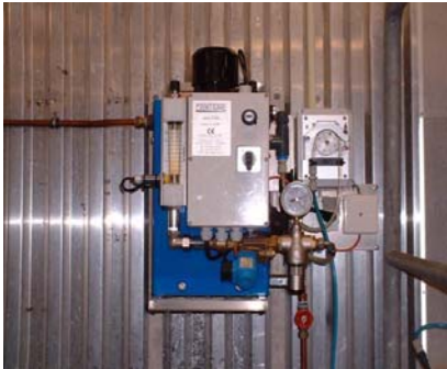
Polymore: Polymer dosing unit. Liquid polymer and water is mixed. See manual for adjustments.
