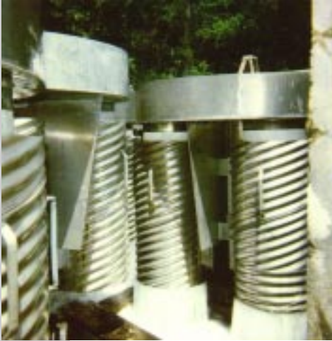
WMT Packed Column, 500 gpm, H 2 S Stripping
