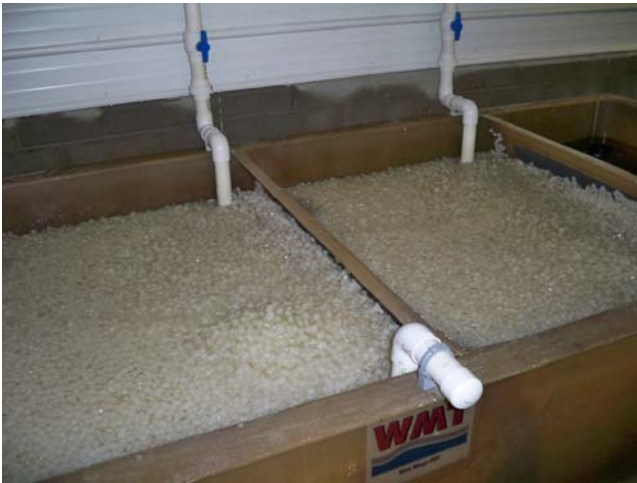
Commercial Tilapia Farms - Mini-IMF Biofilter with Air Grid and Media Screens – 180 gpm, 145 ft 3 media (4.1 m 3 )
