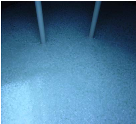
Numana Tribal Hatchery – Custom Biofilter Shell and Media and Media Screens – 2,000 gpm, 500 ft 3 media (14m 3 )
