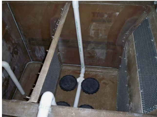
Commercial Tilapia Farms - Mini-IMF Biofilter with Air Grid and Media Screens – 180 gpm, 145 ft 3 media (4.1 m 3 )
