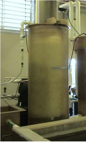
Go Fish GA – Vertical IMF Biofilter with Air Grid and Media Screen – 6 systems (60-180 gpm), 15-75 ft 3 media (0.42-2.1m 3 )
