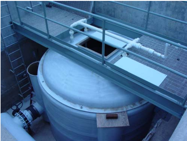
Numana Tribal Hatchery – Custom Biofilter Shell and Media and Media Screens – 2,000 gpm, 500 ft 3 media (14m 3 )
