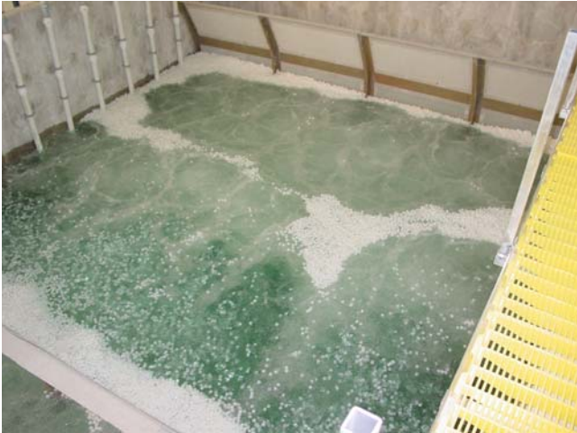
Commercial Trout Farm - Mega-IMF Biofilter with Air Grids and Media Screens – 5,400 gpm – 4,000 ft 3 media (113m 3 )
