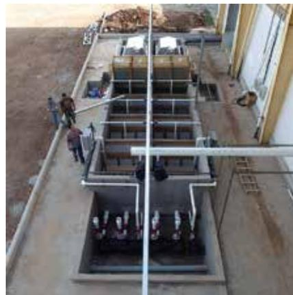
The **Horizontal IMF** was developed to deliver a scalable, low head modular filtration solution. The Horizontal IMF can be applied to intake, RAS, or effluent polishing applications.
